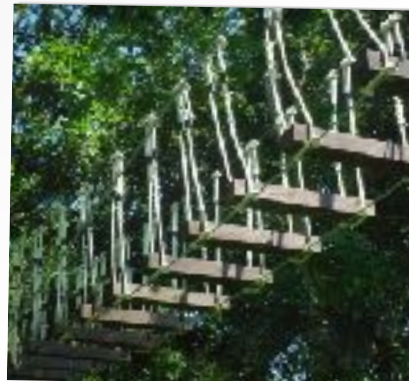
HIGH ELEMENT INSPECTION
