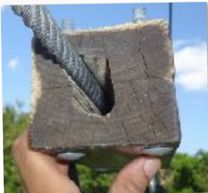
VISUAL & TACTILE INSPECTION
