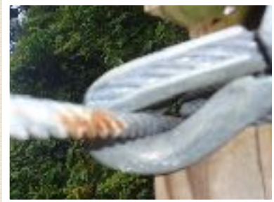
WIRE CABLES INSPECTION
